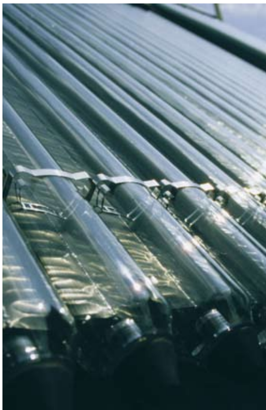
Figure 8.1 Evacuated tube collectors
