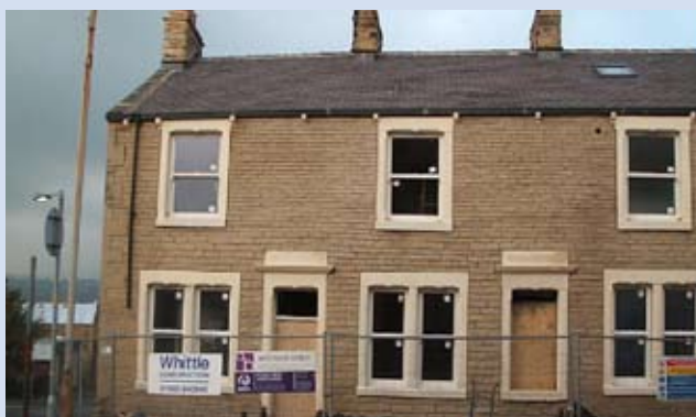
Refurbishment nearing completion
